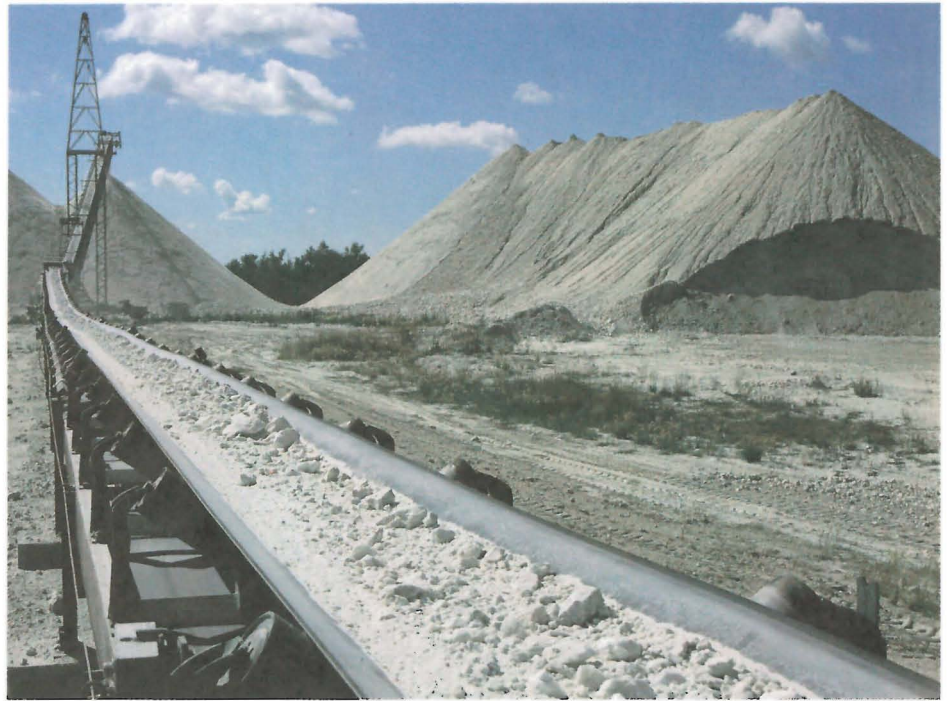
Silica sand conveyor belt and raw material storage, Black Island.
