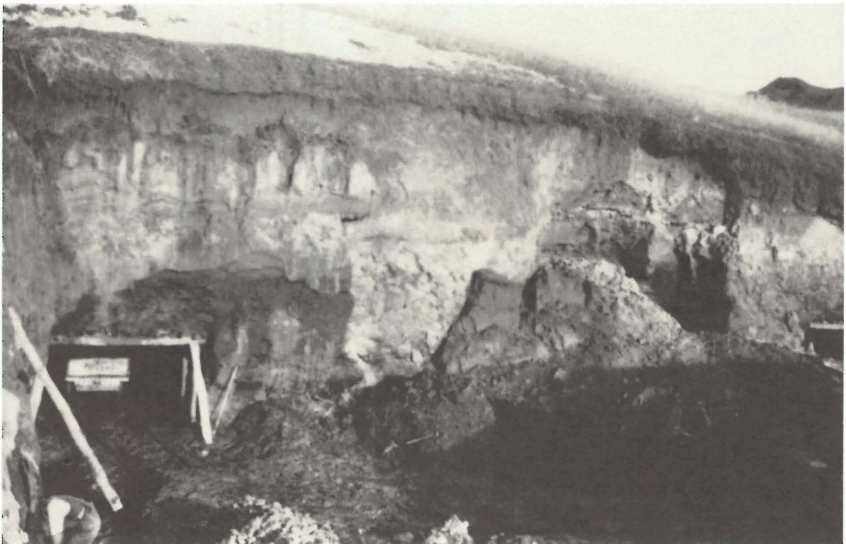
Plate 2. An adit for lignite on the western slope of Turtle Mountain.
