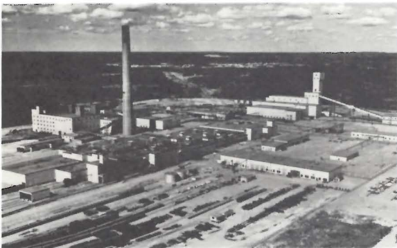
Photo 68. T-1 Mine Plant Area, Inco Metals Company, Thompson (INCO).
