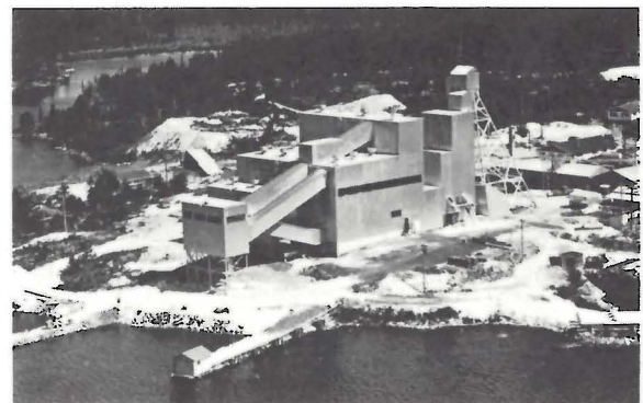
Photo 80. Surface Plant, TANCO Mine, Bernic Lake (MED).
