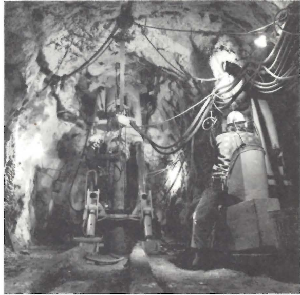
Photo 72. Raise Boring Machine at an Inco Metals Company Mine, Thompson Area. The raise is bored to its full size to provide access from one level to another (INCO).
