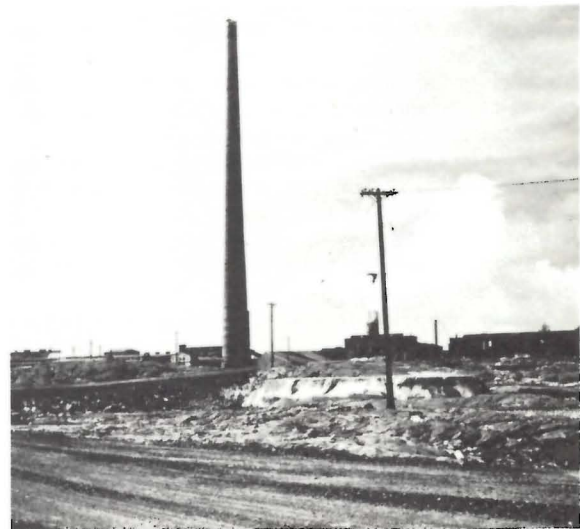
Photo 45. Flin Flon Smelter, H.B.M. & S. Construction of new stack completed, 1973 (MRD).
