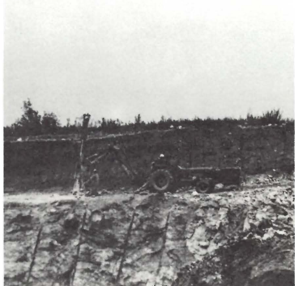
Photo 23. Quarrying Gypsum at Harcus, Western Gypsum (1978) Limited. Drilling the Bench.
