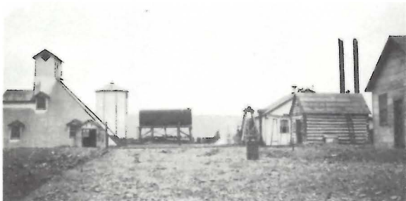
Photo 39. Surface Plant, Mandy Mine, Mandy Mining Company, Flin Flon Area, 1929. Manitoba's first base metal producer (MRD).
