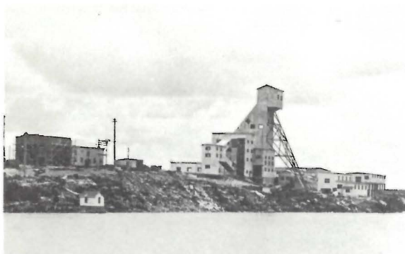
Photo 52. Surface Plant, Sherridon Mine, Sherritt Gordon Mines Limited, Sherridon, 1932 (MRD).
