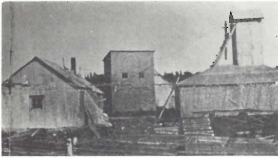
Photo 77. Jack Nutt Shaft and Power Plant, Jack Nutt Mines Limited, Bernic Lake (ca. 1930) (TANCO).
