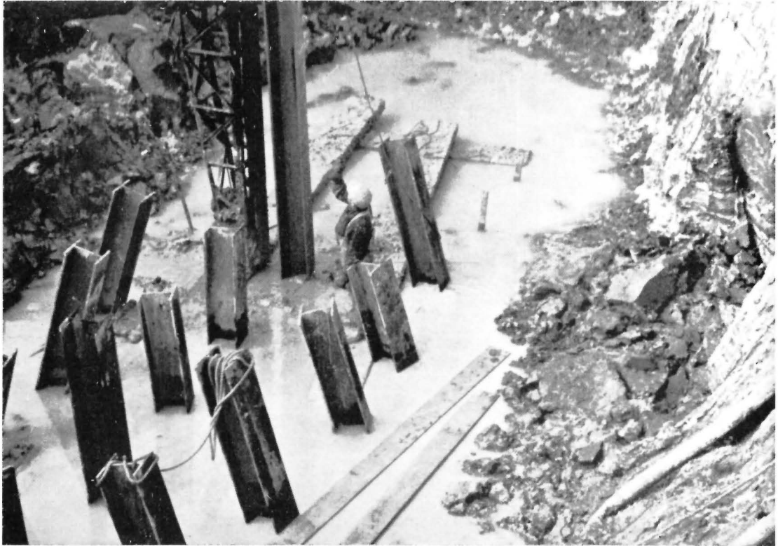
FIG. 21. Pier excavation at the C.P.R. Keewatin Bridge.
