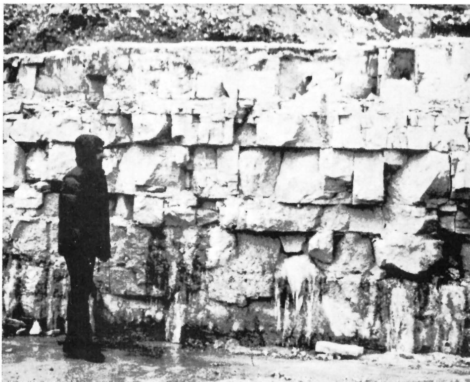
FIG. 10. Upper bedrock zone under the Red River Floodway Inlet control structure.
