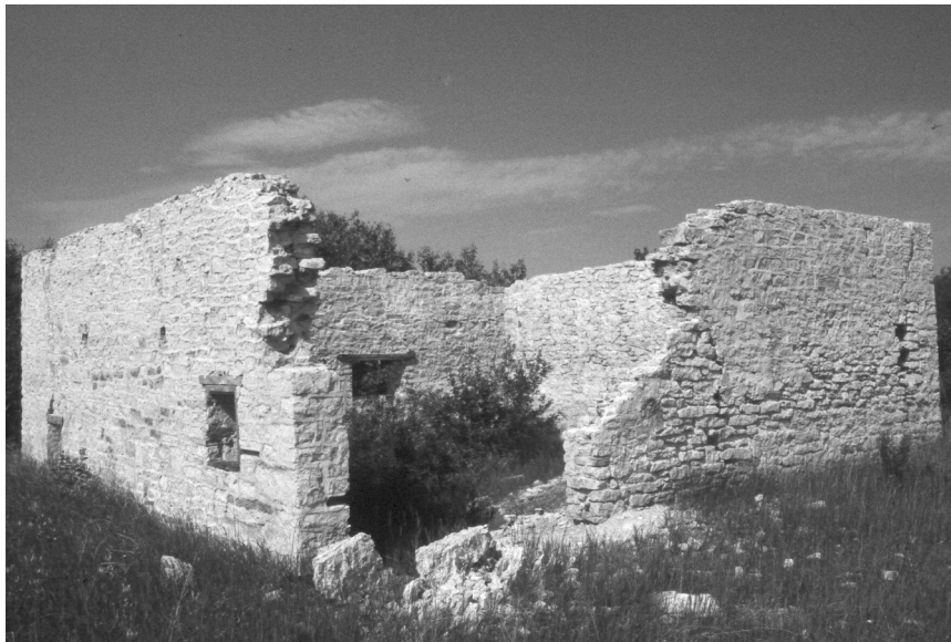
Figure 21: a) Kiln remnants at the northeast end of the Gunn or No. 2 Quarry, next to the railway track. The Gunton Member of the Stony Mountain Formation was used to construct the kiln walls. b) Remnants of a structure near the south end of the Williams or No. 1 Quarry, near the railway track. The Gunton Member of the Stony Mountain Formation was used to construct the walls.
