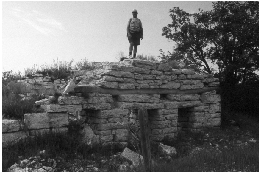
Figure 21: a) Kiln remnants at the northeast end of the Gunn or No. 2 Quarry, next to the railway track. The Gunton Member of the Stony Mountain Formation was used to construct the kiln walls. b) Remnants of a structure near the south end of the Williams or No. 1 Quarry, near the railway track. The Gunton Member of the Stony Mountain Formation was used to construct the walls.
