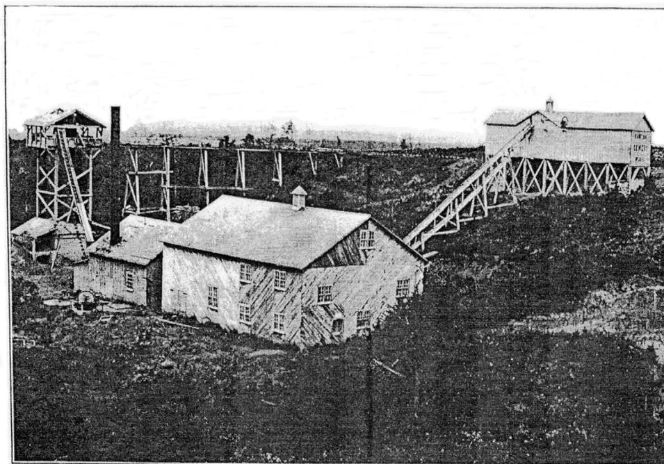
VIEW OF ARNOLD CEMENT WORKS, PEMBINA HILLS, SHOWING VERTICAL CLINKER KILN, CLINKER GRINDING HOUSE AND STORAGE SHED ON THE CANADIAN NORTHERN RAILWAY.
