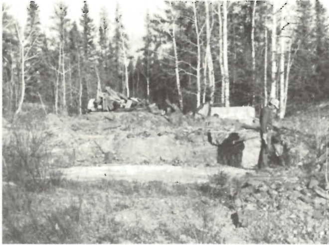
Concrete footings and capped shaft at the Gold Lake property. Field trip stop #5.
