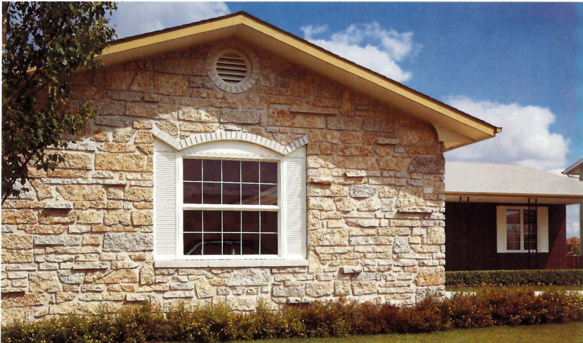
Mixed Buff and Grey Rustic Ranch Rock Coursed Pattern with some projecting pieces. Note cut stone window sill and trim.
