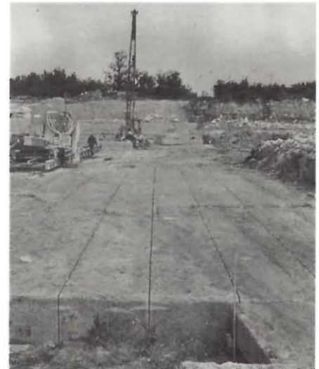
Quarrying Tyndall stone near Garson. Straight lines were cut using tungsten carbide-toothed circular saw.
