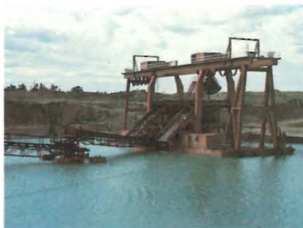
Floating twin clam-shell excavator operating in Birds Hill gravel deposit, 1982.
