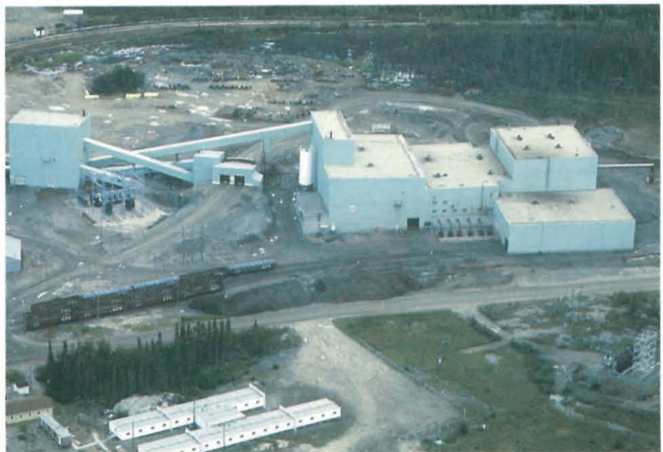
Aerial view of the Stall Lake concentrator of Hudson Bay Mining and Smelting, 1986.
