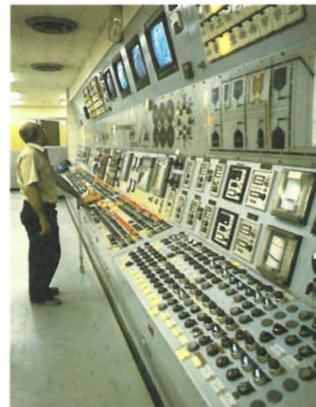
Control room in Inland Cement's plant at Fort Whyte, 1987.
