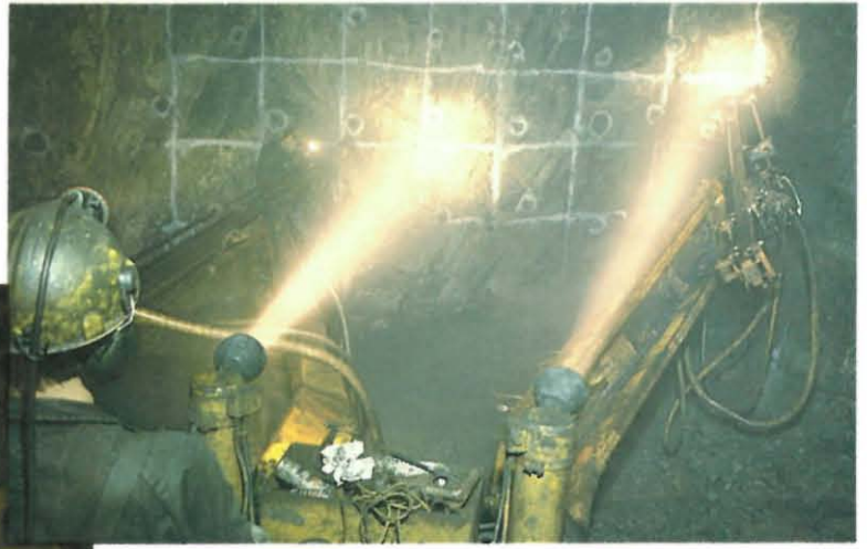
Drilling the working face for setting of explosives at Sherritt's Ruttan Mine, 1986.
