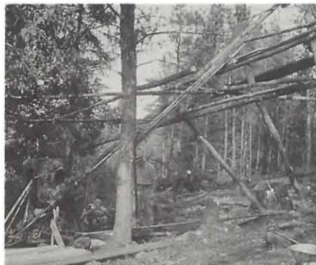
Drill set-up on the Sunbeam-Waverley gold prospect, 1944 (Provincial Archives).
