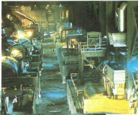
Far Right: Crushing and grinding ore in mills at Inco's Thompson concentrator, 1980.
