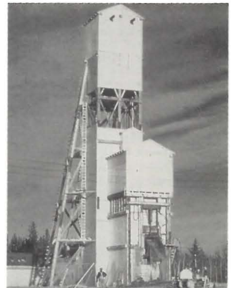
Inco's Thompson mine original development shaft (T-2), 1956.
