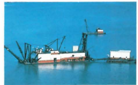
Dredge at work removing mud and muskeg above "crown pillar" of the Thompson orebody, 1983.
