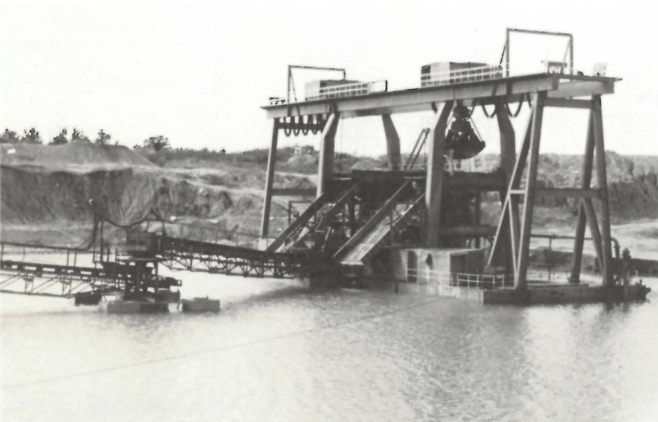
Figure 18: A floating twin clam-shell excavator in operation in the Birds Hill gravel deposit. The sand and gravel is excavated from depths of up to 20 metres and transported to shore for final processing by a floating conveyor system.
