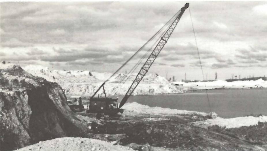
Figure 17: Dragline excavating gravel from below the water table in the Birds Hill gravel deposit.
