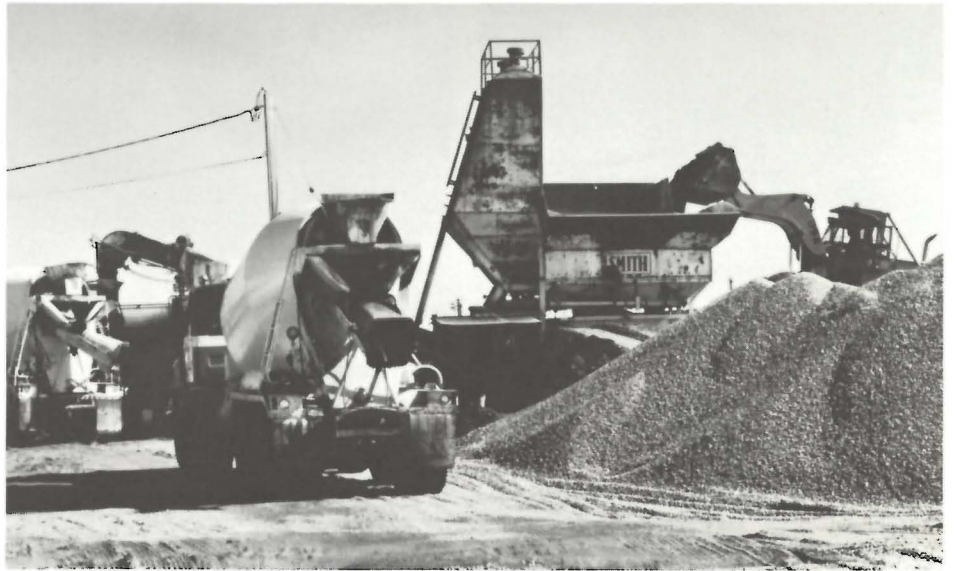
Figure 9: Stockpiled gravel is blended to form concrete at a portable concrete plant, then is loaded and trucked to the work site.
