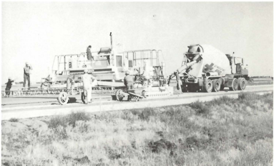
Figure 10: Concrete is poured and spread on a gravel base for a new highway.
