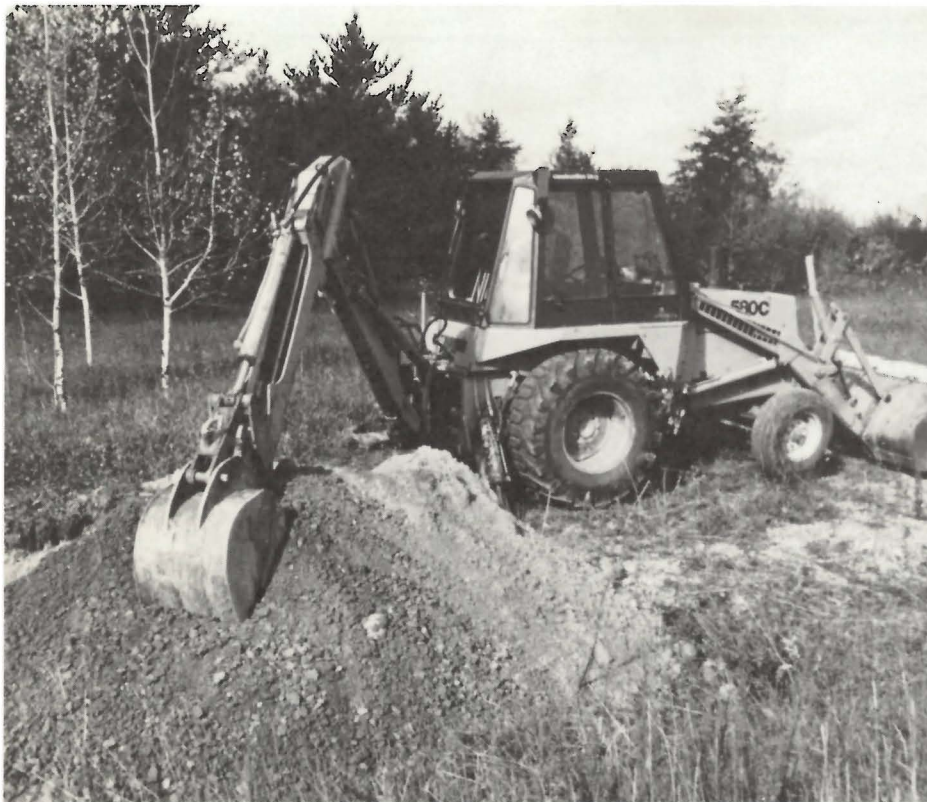
Figure 14: Testing a potential sand and gravel source with a backhoe.
