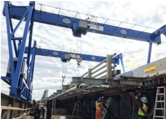
Figure 1: Overhead Gantry Crane in operation
