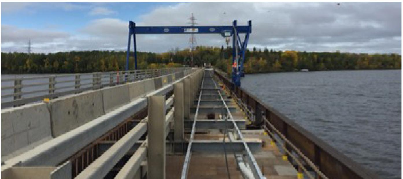
Figure 2: Overhead gantry crane system utilized for demolition and erection of the new structure
