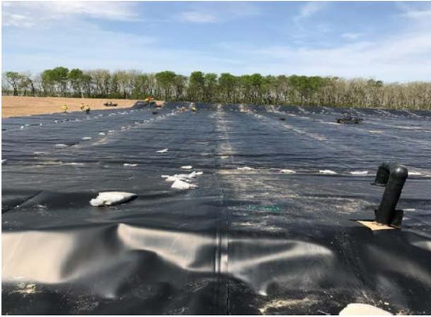
**Grand Beach Lagoon Installing Liner on Secondary Cell**
