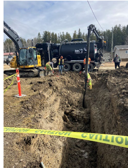
Bissett Water & Sewer Renewals
