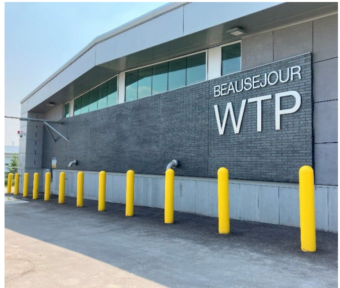
Town of Beausejour Water Treatment Plant
