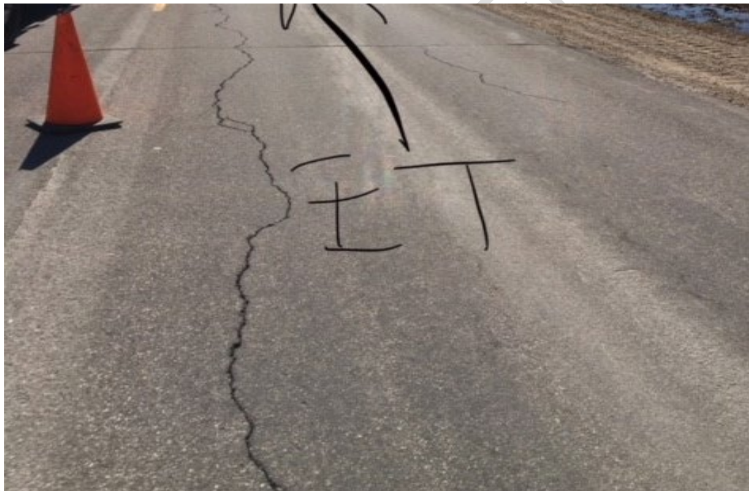
Figure 2.0.5: Longitudinal Cracking on PTH 67 at PTH 8, Manitoba
