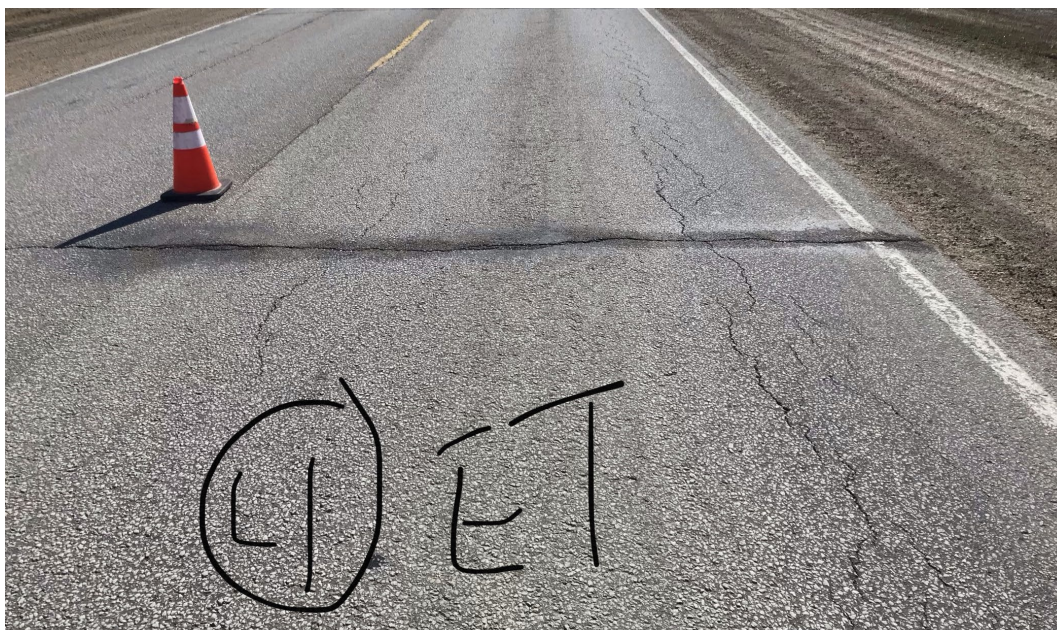
Figure 2.0.4: Bottom- Up Fatigue Cracking in Wheel Path on PTH 2 at Oak Bluff, Manitoba
