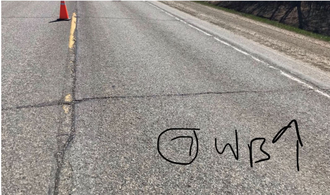
Figure 2.0.6: Transverse Cracking on PTH 23 at Carmen, Manitoba
