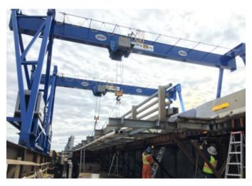
Figure 1: Overhead Gantry Crane in operation
