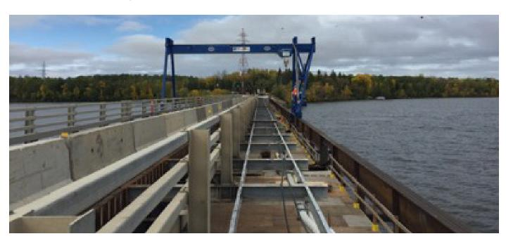
Figure 2: Overhead gantry crane system utilized for demolition and erection of the new structure
