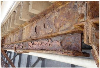
Severe deterioration of the exterior beam on north side
