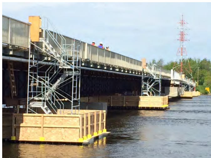
Bridge construction site
