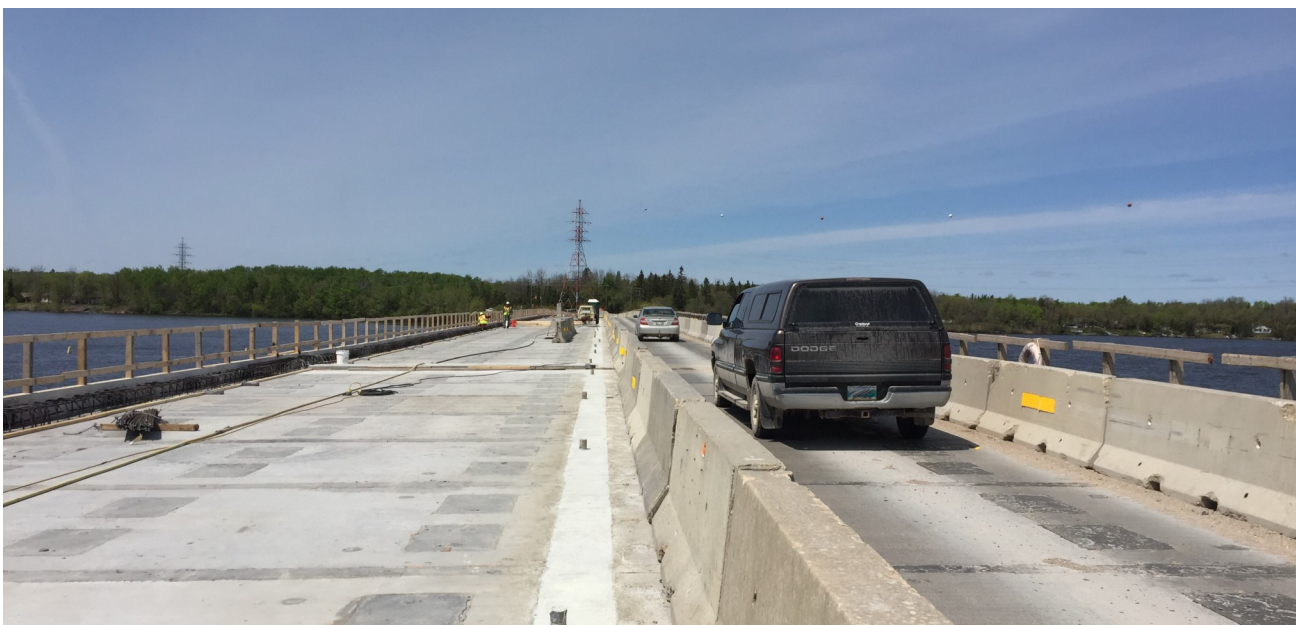
Figure 2: South lane of bridge construction nearing completion
