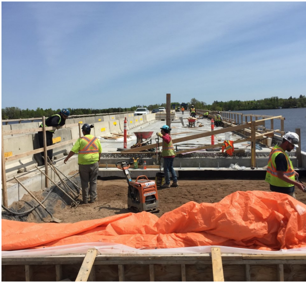
Figure 1: Construction of Bridge approach roadwork
