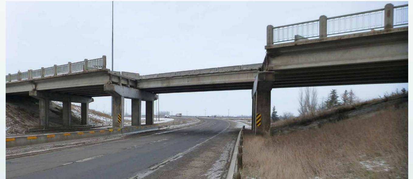
Over the years, **the bridge has been damaged by several vehicle impacts**, and many bridge elements are exhibiting significant deterioration. As a result, the bridge is currently restricted to a single lane.
