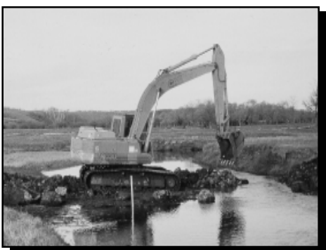
Riffle Construction
