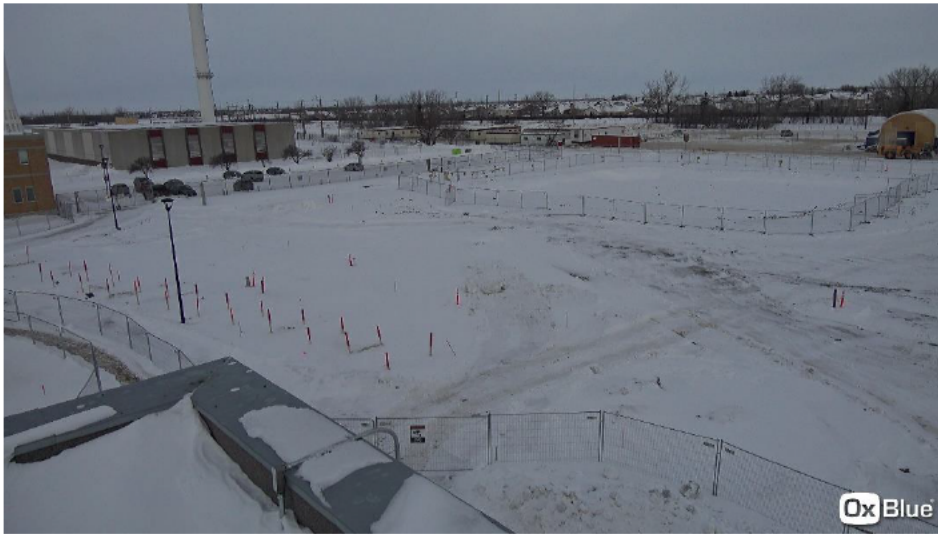
Grit Building Excavation
