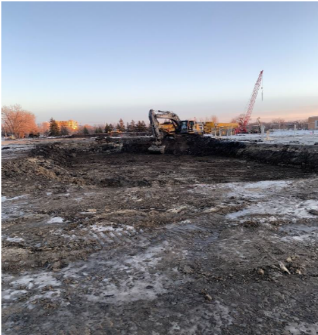
Excavation of Grit Building
