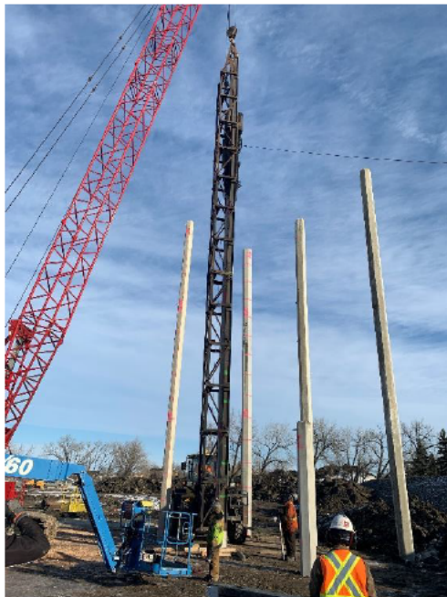
Test Pile Installation
