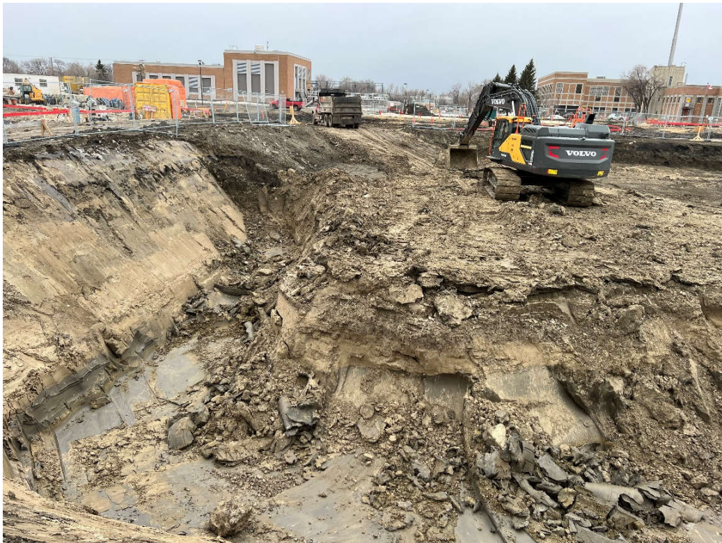
Figure 2: Excavation of Grit Building
