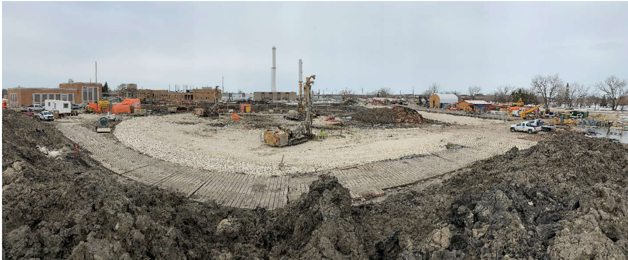
Figure 1: Main Site Overview
