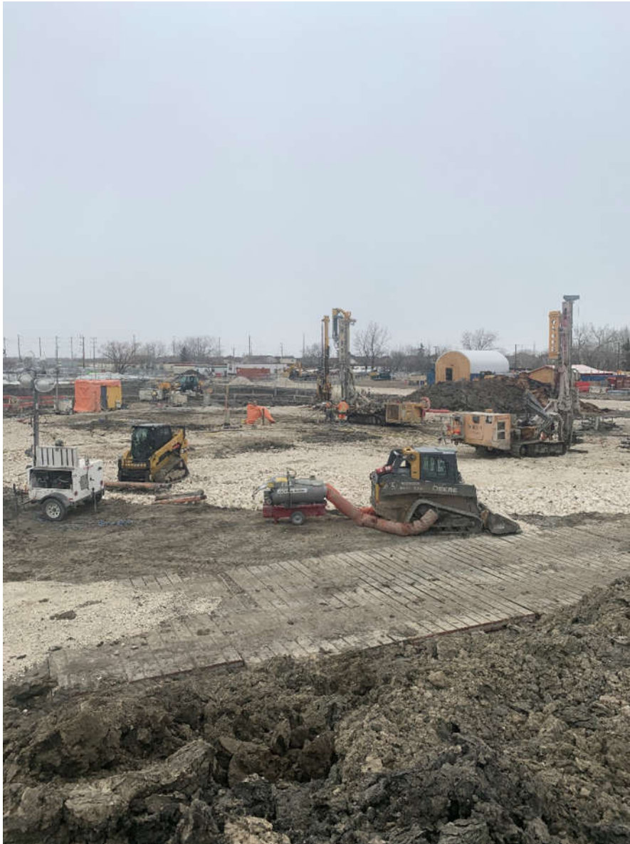
Figure 3: Drilling and Grouting at H2 Area
