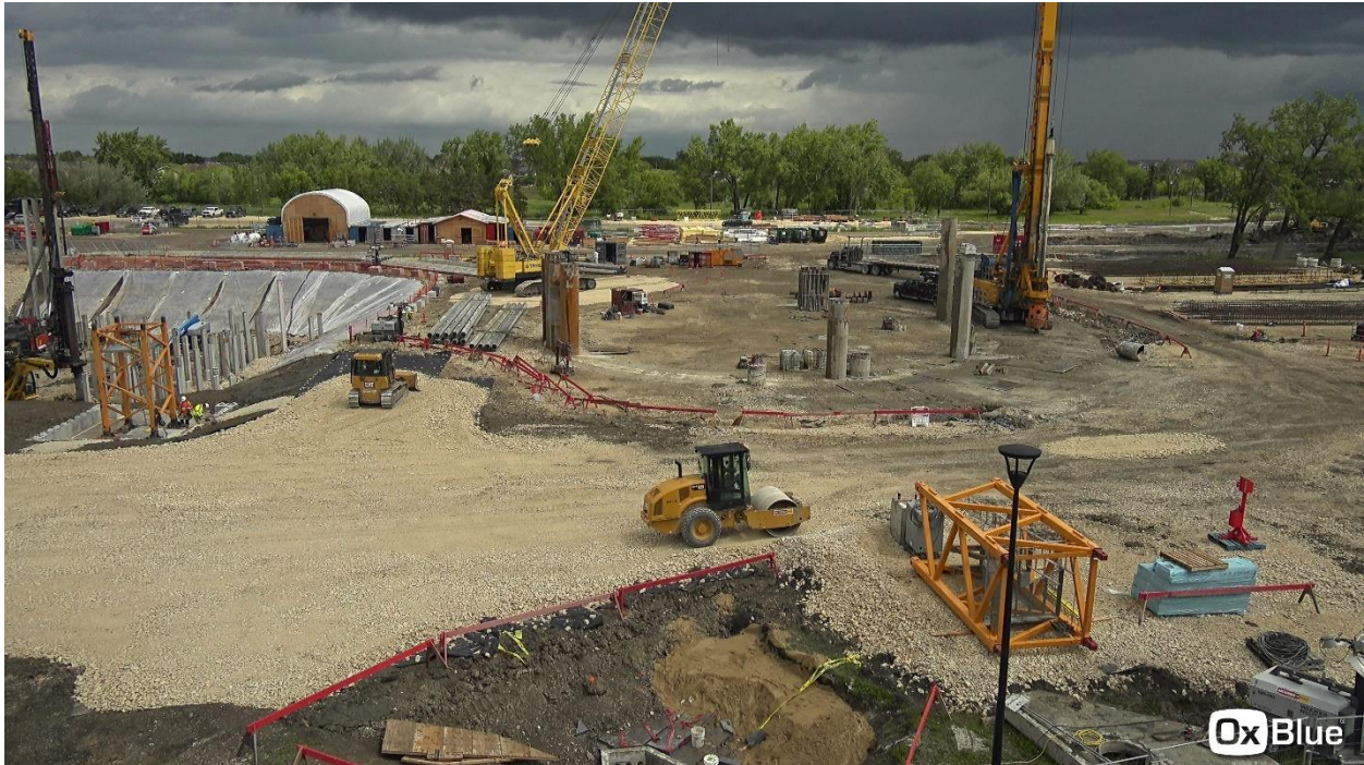
Figure 1: Secant Pile Installation for Pump Station
