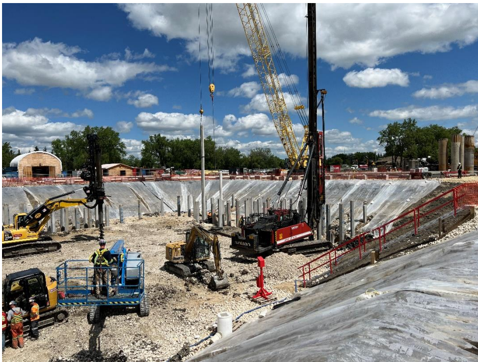
Figure 2: Excavation of Grit Building
