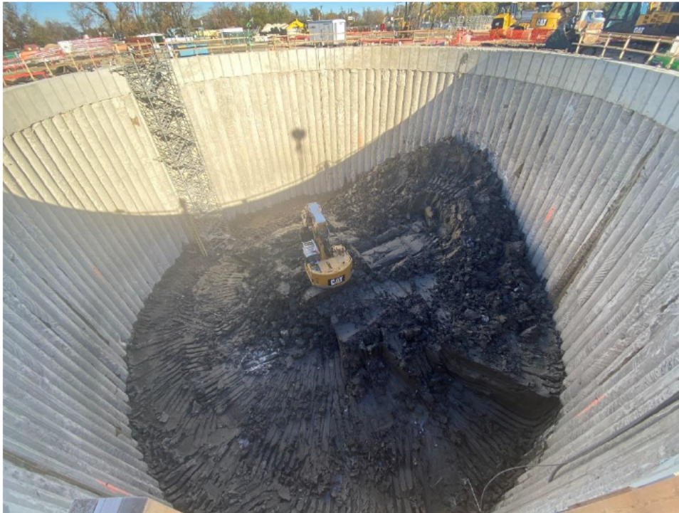
Figure 1: Shaft Excavation for Pump Station
