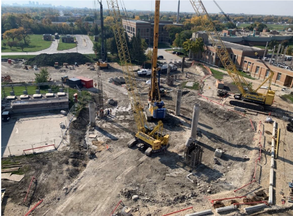
Figure 3: Secant Pile Installation at H1 Area
