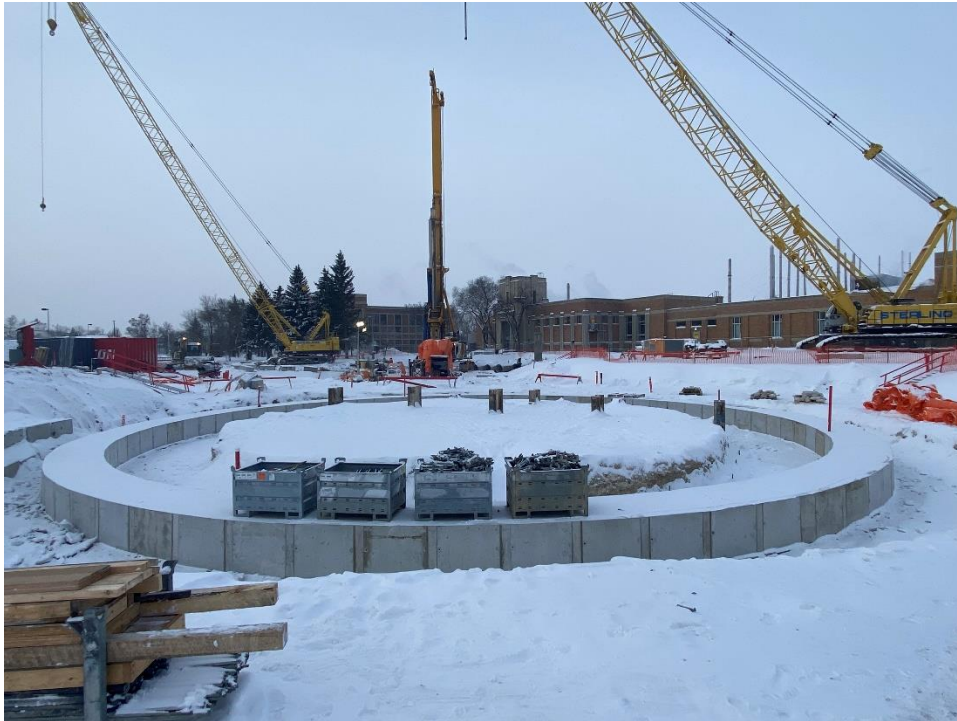
Figure 1: Secant Piles and Ring Beam at H1 Area
