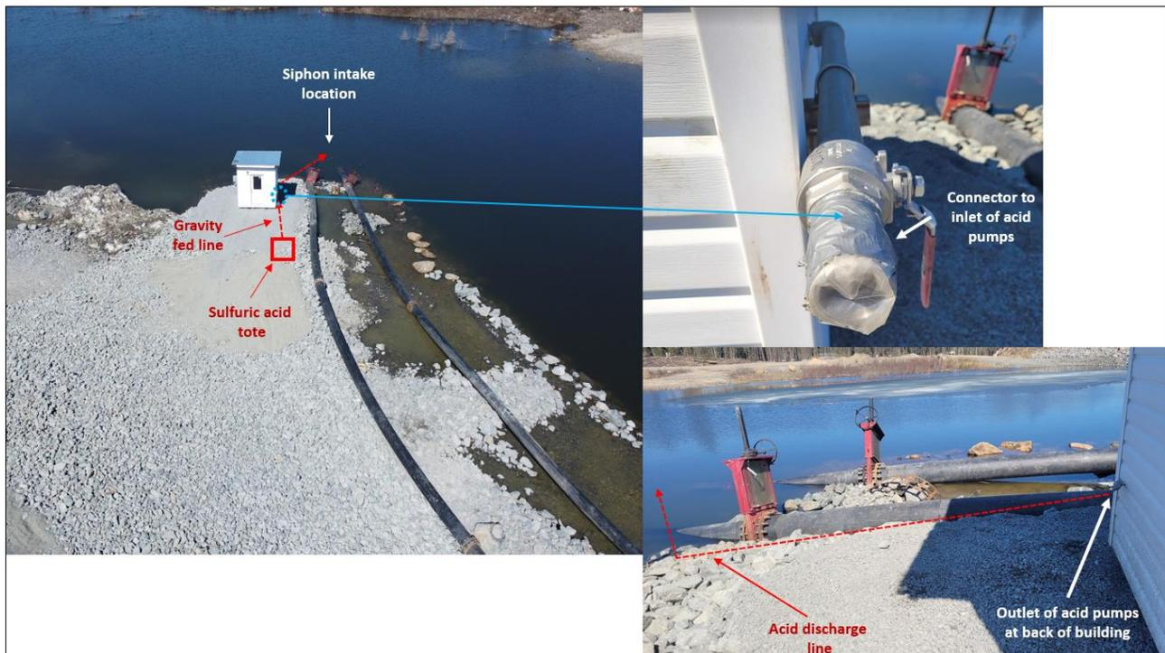
**Figure 3 – Location and Components Acid Dosing Building**
