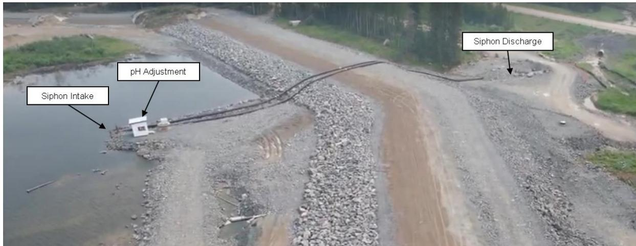
**Figure 2 – Siphon Intake Location and Discharge Location**
