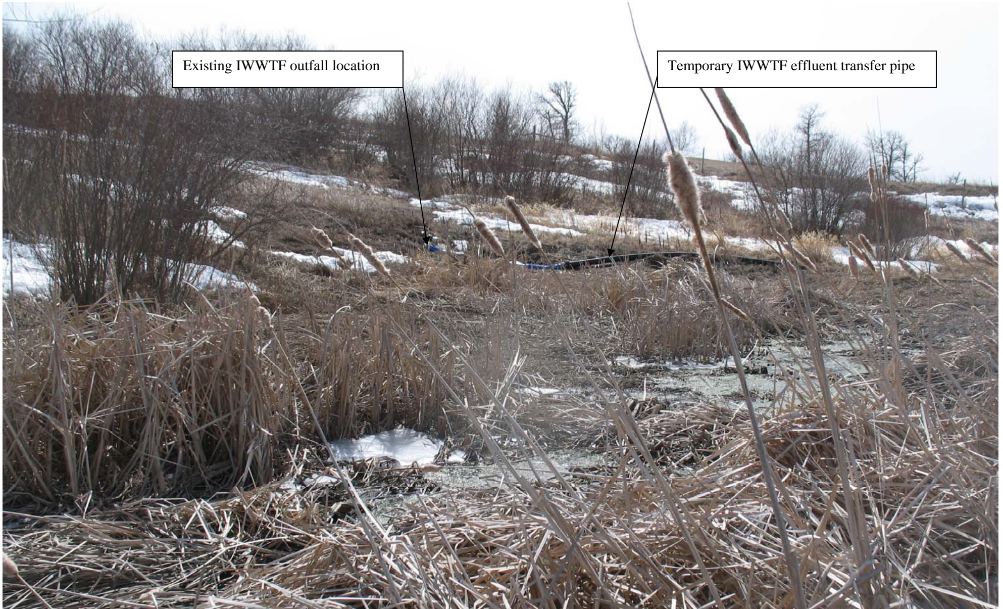
Figure 3.5: IWWTF Outfall Location – Southwest – Facing southwest towards the existing IWWTF outfall location and the temporary IWWTF effluent transfer pipe.
