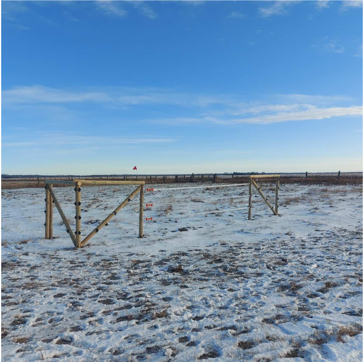
C4: Photo of RTBF trail site, October 26, 2022, fencing around site installed.
