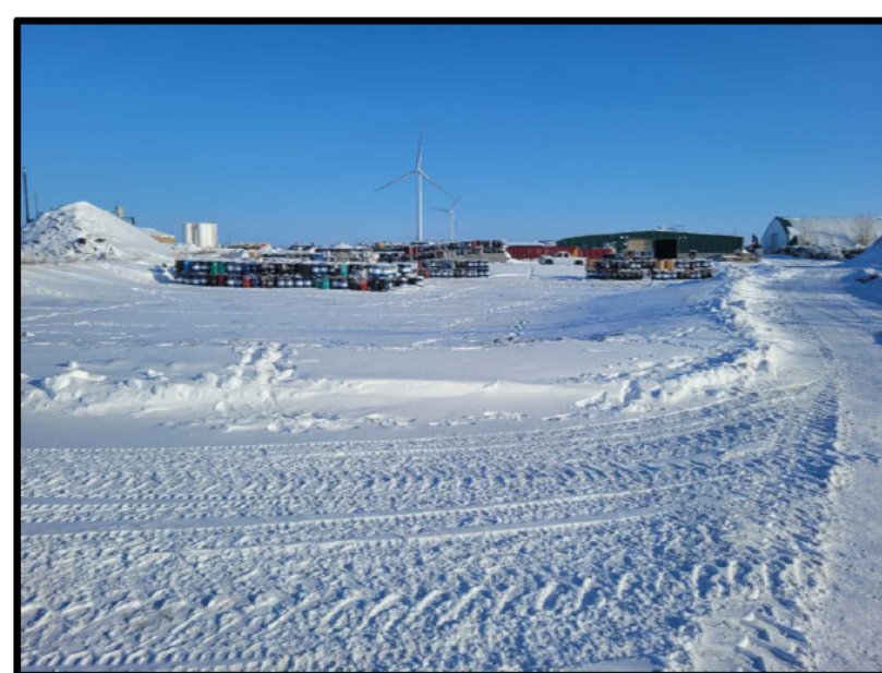
PHOTOGRAPH 3: FACING EAST, SHOWING SOUTH AND WEST BERM
