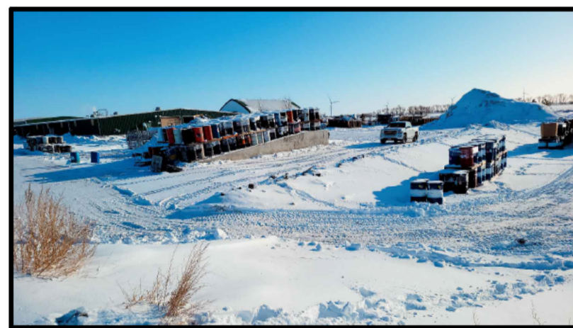
PHOTOGRAPH 1: FACING SOUTHEAST, SHOWING EAST BERM AND VEHICLE ENTRANCE
