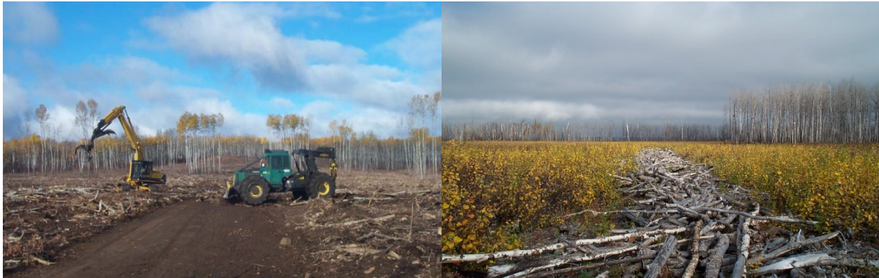
Figure 2.8 Road decommissioning being carried out in a harvest block (left); decommissioned road (right).
