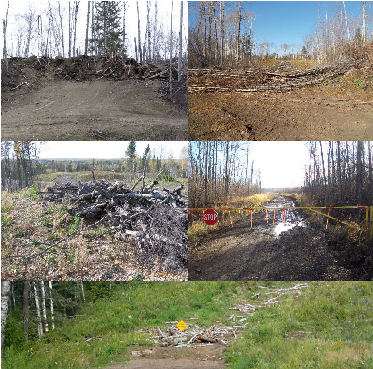
Figure 2.7 Access management examples including road closures or crossing removals.
