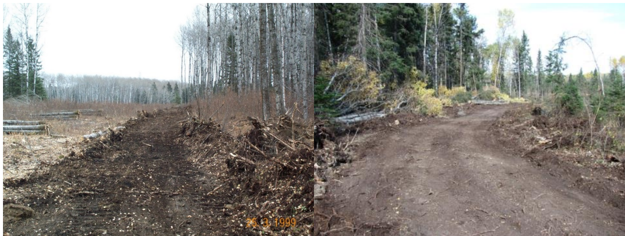
Figure 2.5 In-block road construction.
