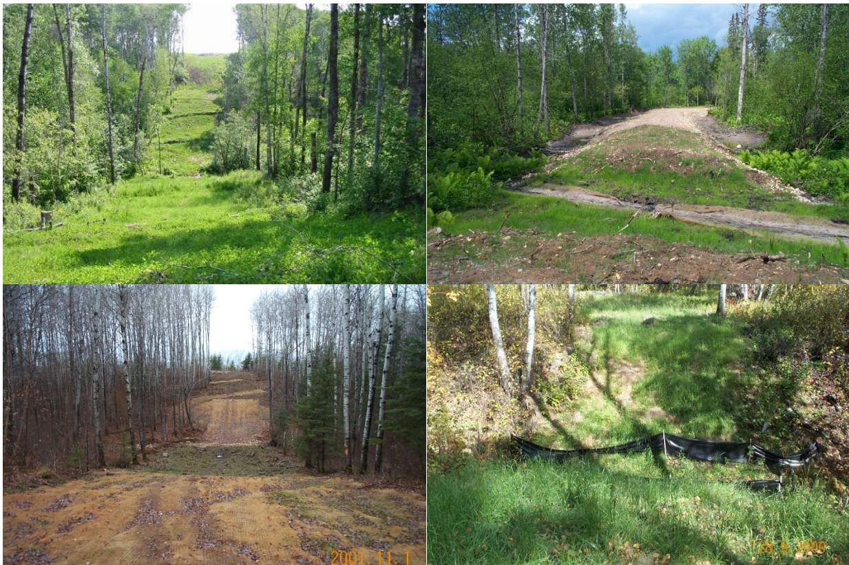
Figure 2.10 Water crossing decommissioning examples.
