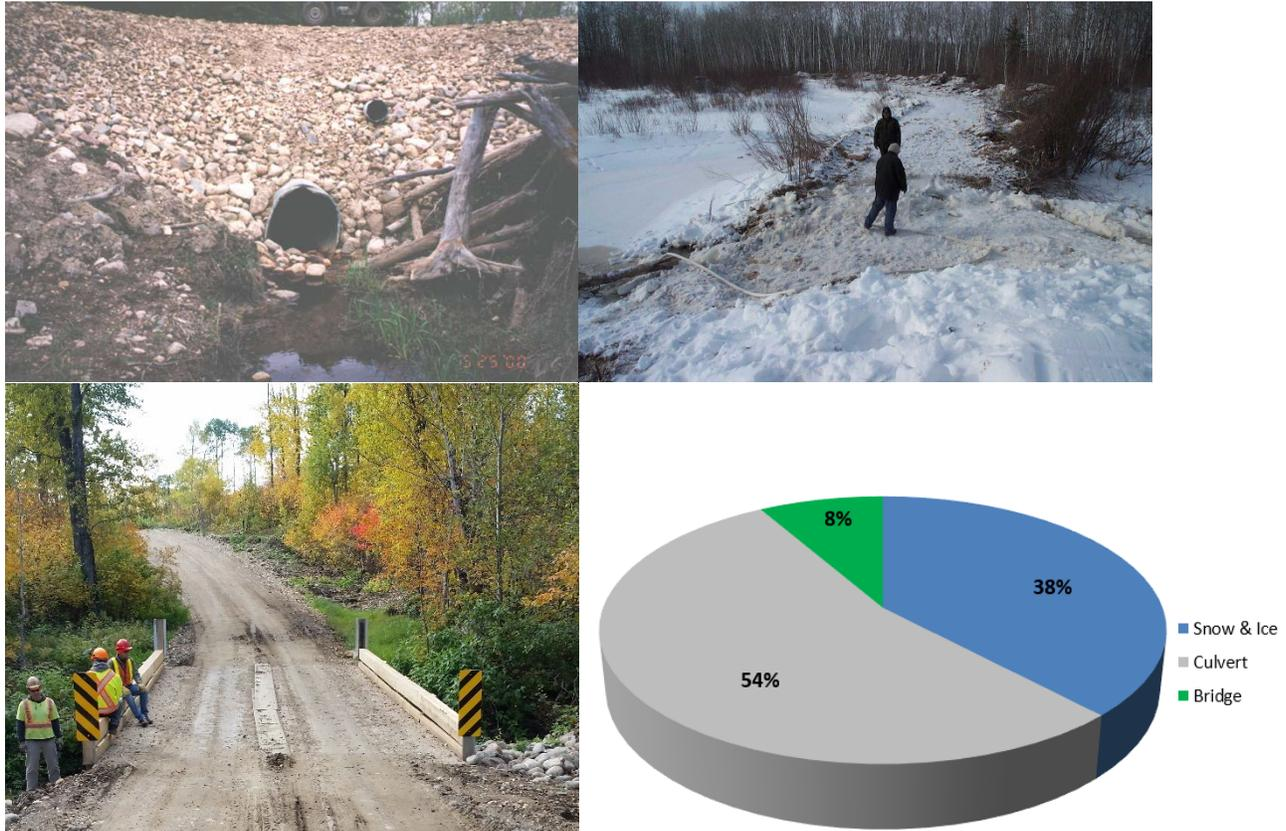
**Figure 3-1: Examples of crossings - round culvert, snow and ice, portable steel bridge, and the percentages of each proposed crossing type.**
