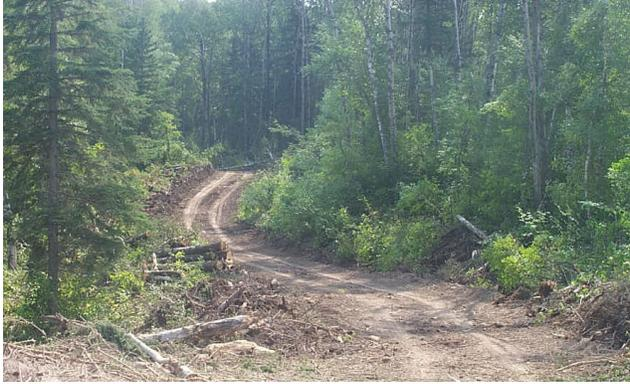
The development of road Right of Ways (ROWs) is an important component of road construction. During summer harvesting, road ROWs are built wider (typically 20 m) to dry the roads quicker by maximizing air movement and sunlight. During winter operations, right of ways can be narrower (typically 15 m).
