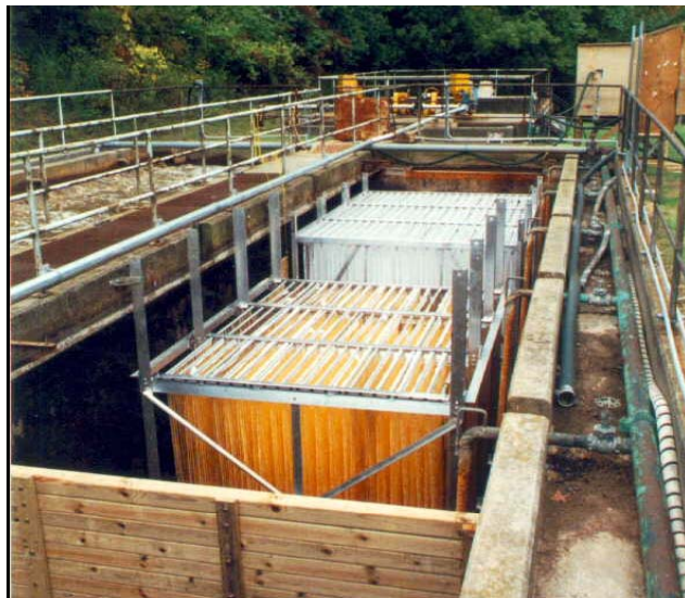
PHOTOGRAPH OF TWO HANGING FIXED MEDIA IFAS MODULES INSTALLED IN A BIOREACTOR AT THE WATERDOWN, ONTARIO WWTP
