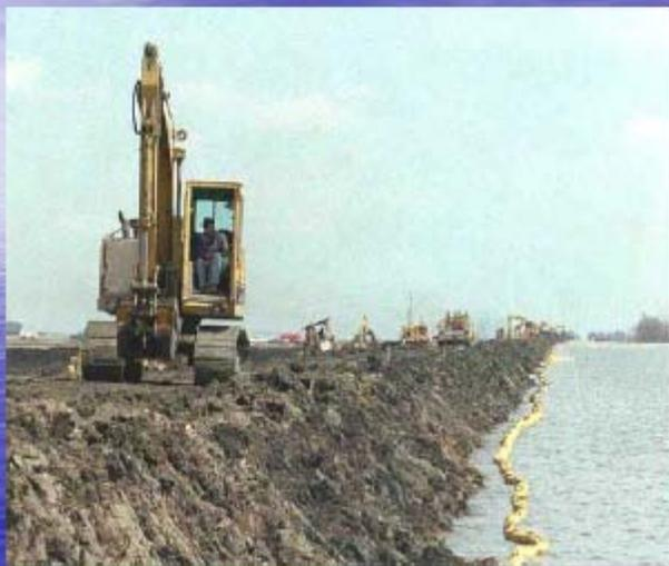
In 1997, the West Dike was expanded on an emergency basis. This dike prevented floodwaters from sweeping west of the floodway and entering Winnipeg from a southwestern flank. Enhancements to this dike would provide additional freeboard and wave protection for this structure.
