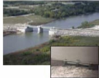
Floodway Gate Control Structure shown (top) under normal water levels, and (right) during 1997 Flood operations.
