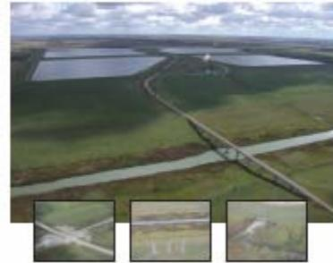
The Floodway Channel is crossed by bridges (top), roads, hydro transmission lines, drainage structures and other crossings. Most of these crossings require modification.
