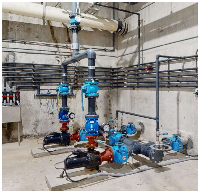
Figure 4-1: WAS Pump Current Piping Configuration
