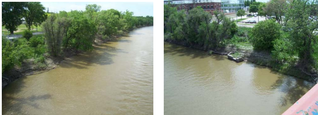
Figure 6.5a-b South bank looking: (a) downstream west of and (b) upstream east of existing river bridge (Dillon 2009)
