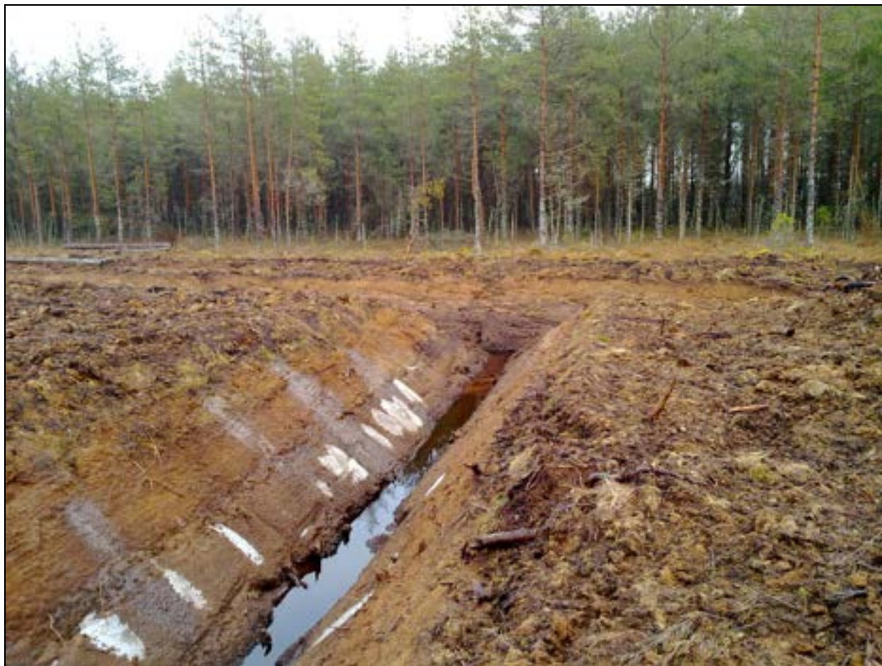
Figure 3 Photo of a Main Ditch
