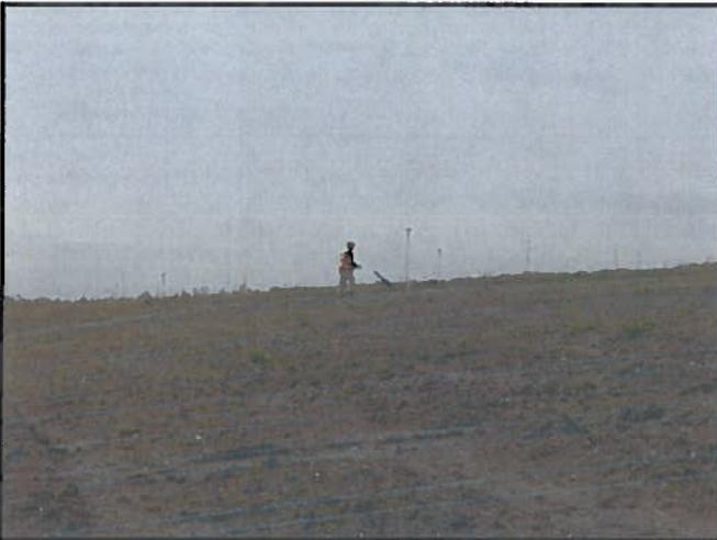
**Photograph 2:** A cap of fabricated biosolids soil mixture placed on a portion of the Ecowaste landfill, prior to vegetation establishment, Richmond, B.C.
