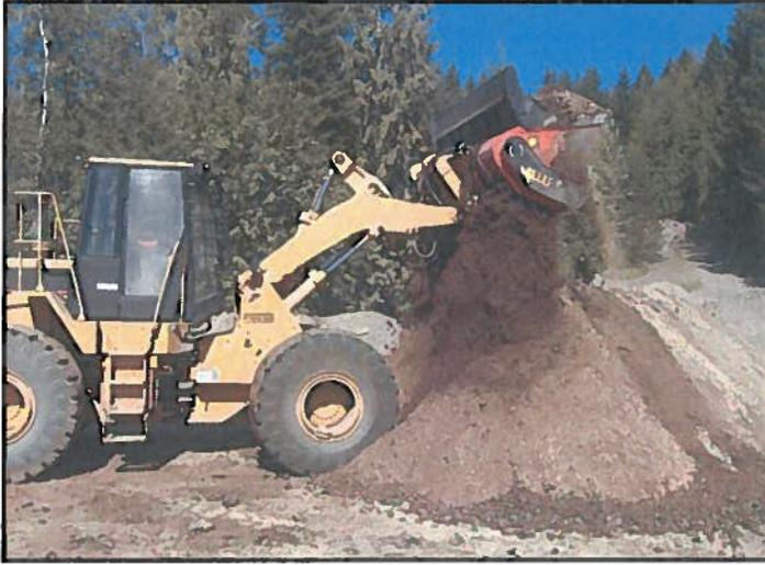
**Photograph 4:** Soil feedstocks are combined with an ALLU bucket to fabricate a biosolids soil mixture, Skimikin Landfill, B.C.
