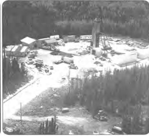
Hoist house and headframe over the Lalor ventilation shaft. — photo courtesy of HudBay Minerals
