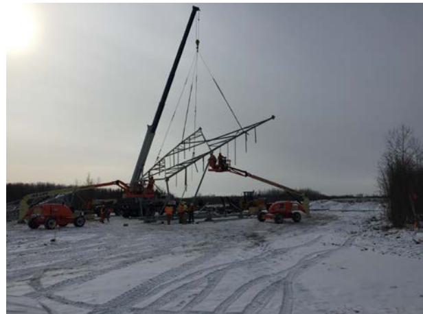
Photo 1: Construction crews installing a tower
