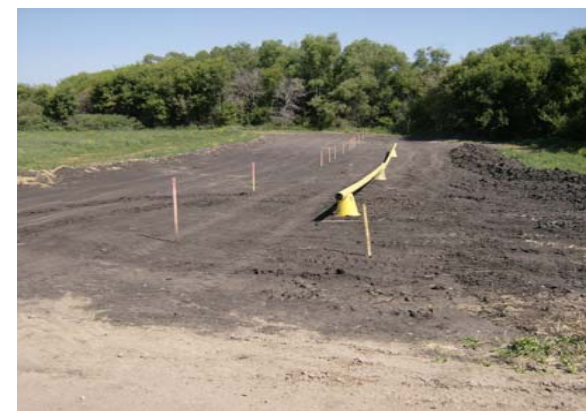
Preparation for trenching and pipeline installation.
