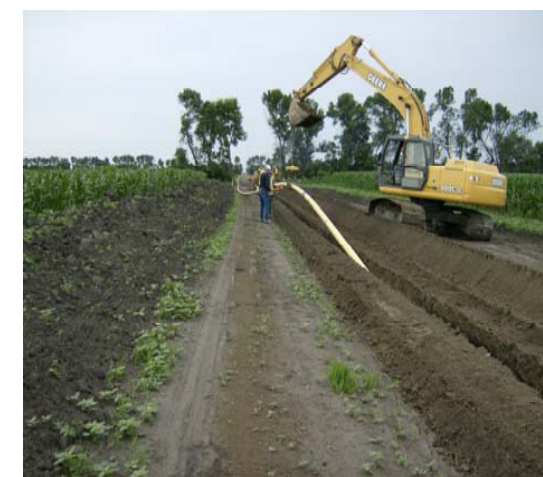
Trenching being undertaken for a past gas pipeline project by Manitoba Hydro
