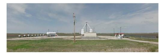
This alignment would require routing the transmission line over an anhydrous ammonia storage facility that is located on PR210 (see also image below), which is not possible due to safety hazards. Note that the tubular steel H-frame tower structure being utilized for road alignment placement in this Project would place the preferred route more than 60m away from the home in question allowing tighter alignment with the road, and minimizing obstruction to in-field operations.
