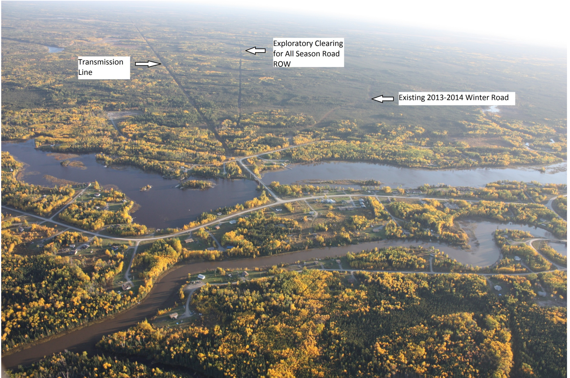
Photo 18: Poplar River First Nation, looking south across Poplar River (Note transmission line right of way, exploratory clearing along proposed all season road alignment, and existing 2013-14 winter road) Photo Credit: Joro Consultants
