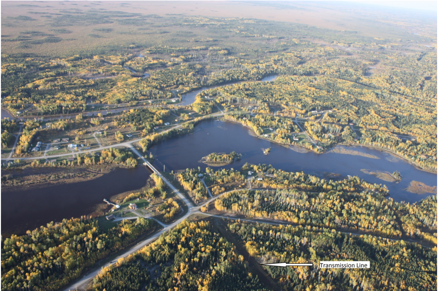
Photo 17: Poplar River First Nation, looking north across Poplar River. Proposed Community Access Road will connect to existing community road network south of bridge. (Photo Credit: Joro Consultants)
