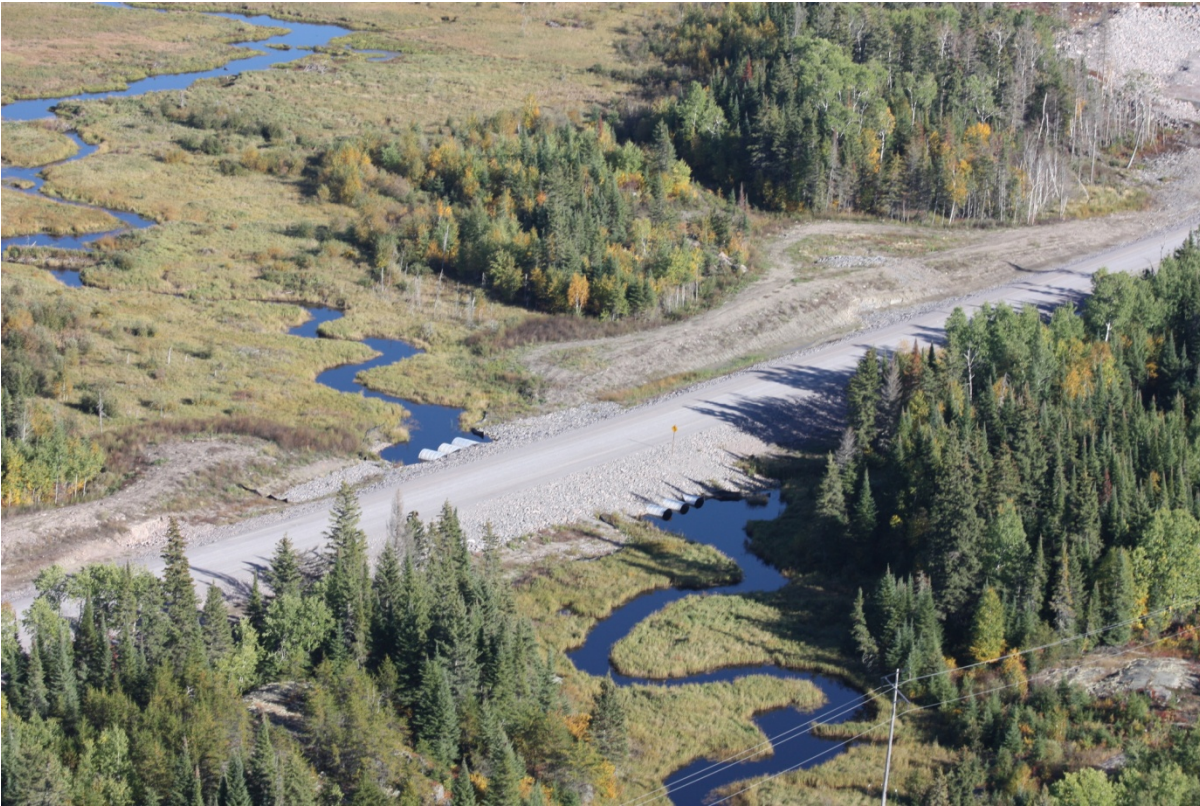
Photo 12: Stream Crossing – Three culverts (representative from P1)
