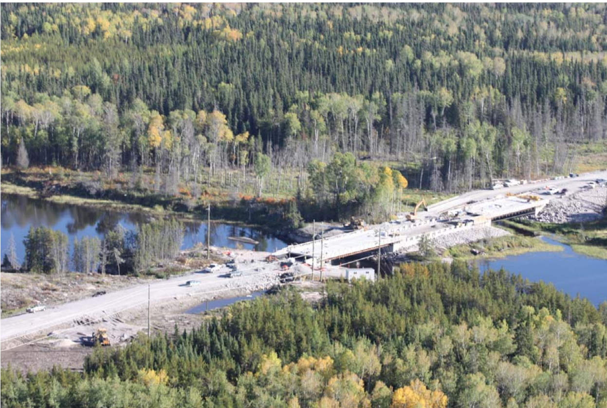
Photo 13: River Crossing – Bridge construction over Bloodvein River (representative from P1)
