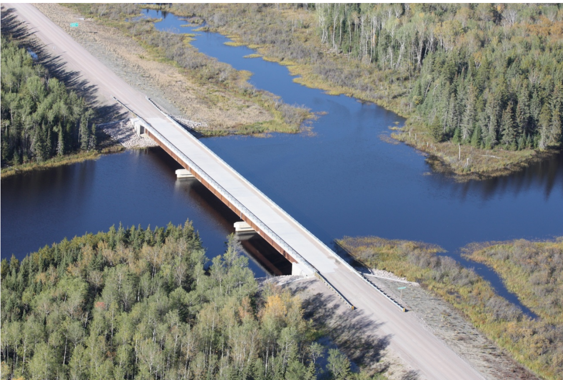
Photo 11: Stream Crossing – Bridge with Piers over Longbody Creek (representative from P1) Photo Credit: Joro Consultants
