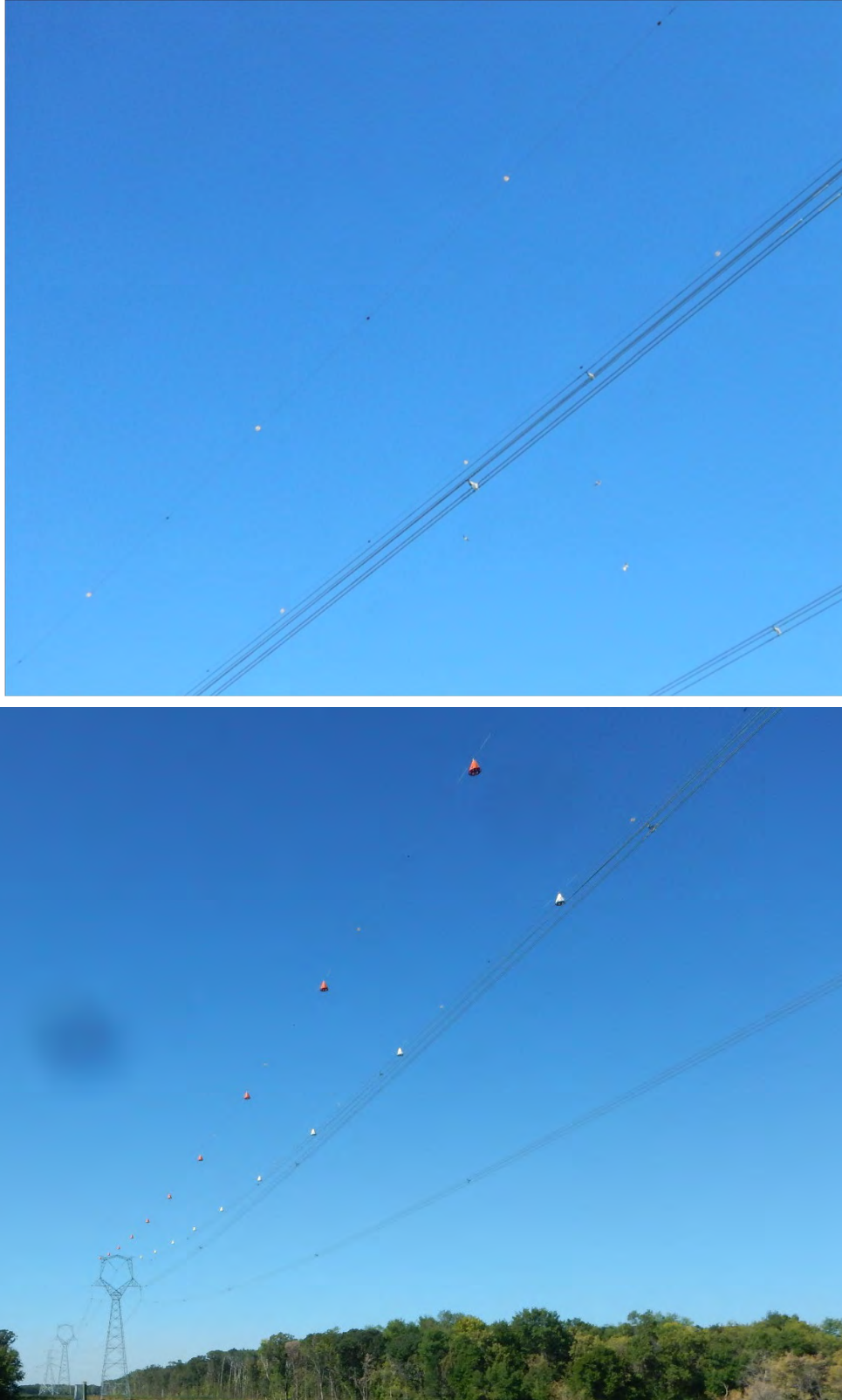
Photo 2. Alternating Swan-Flight Bird Diverters and Bird Flight Bird Diverters (top), and additional aircraft cone markers (bottom) on the Manitoba-Minnesota Transmission Project
