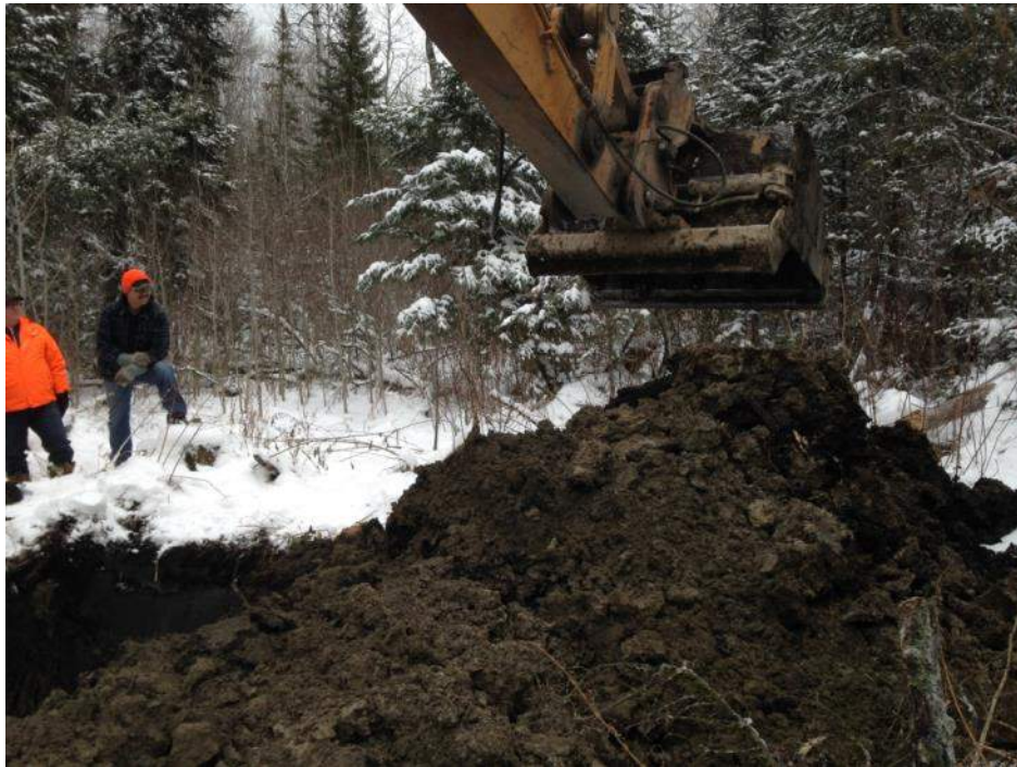
Photo 1. Geotechnical survey at septic field site.
