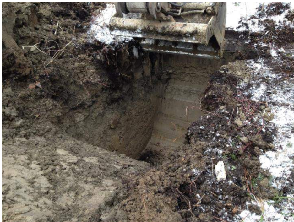
Photo 2. Test pit showing soil profile as part of geotechnical survey.
