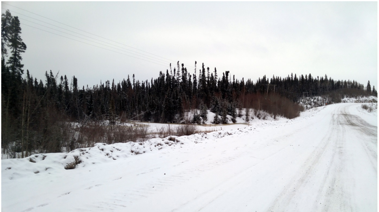
Photo 2: Community access road near abandoned quarry (view: south).
