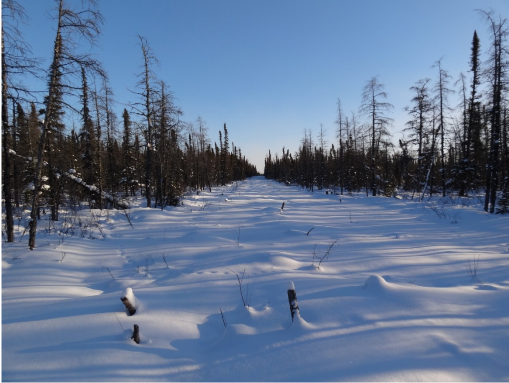
Photo 8: Exploratory clearing completed along proposed All-Season Road alignment approaching Manto Sipi Cree Nation
