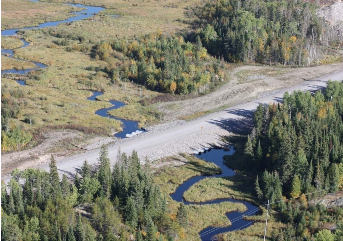
Photo 6: Stream crossing – three culverts (representative from P1)
