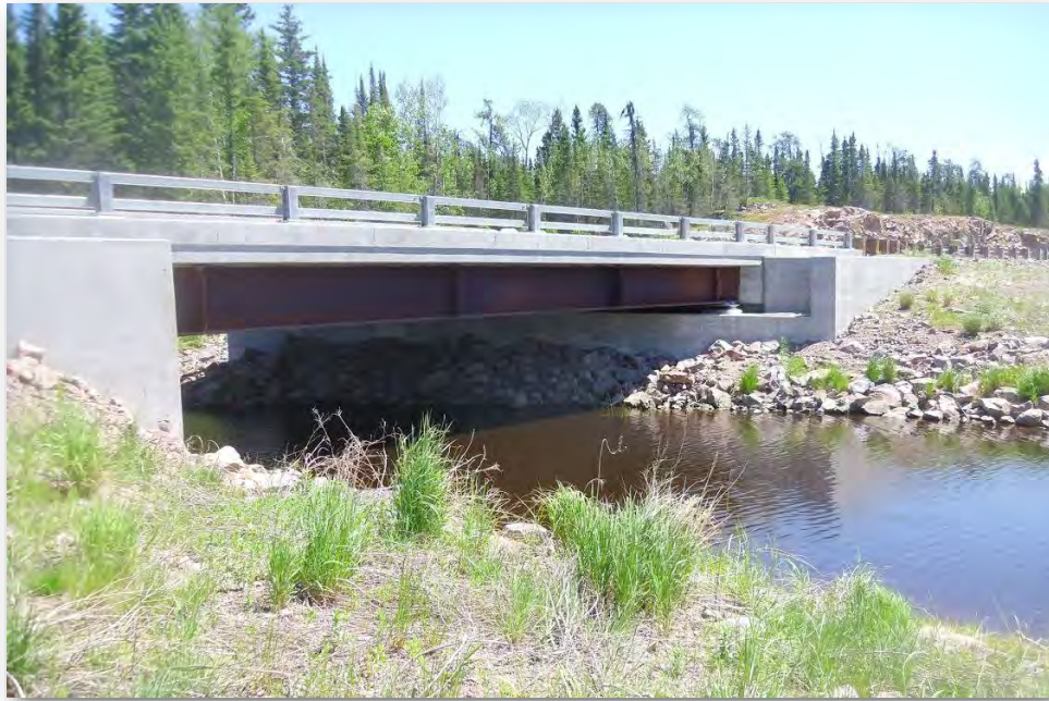
Photograph 3-2: Typical Clear-Span Bridge – Loon Creek (Project P1)
