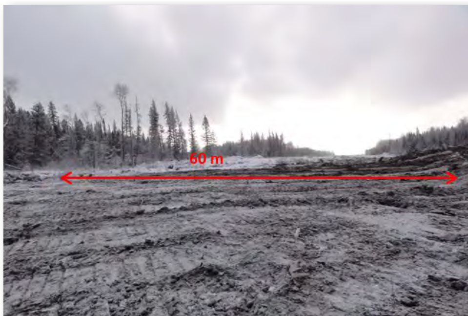
Photograph 3-5: Typical All-Season Road 60 Metre-Wide Right-of-Way Clearing for Construction
