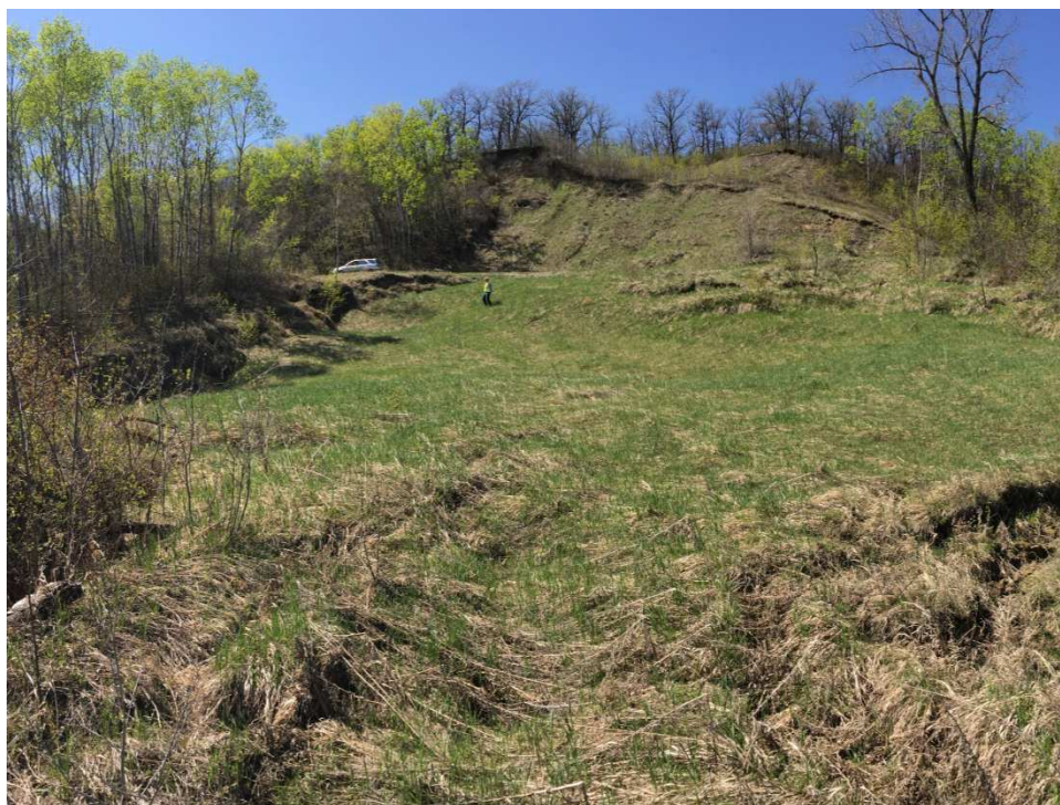
Photo 6 – Bank slip adjacent to road at Site #91 (looking up at road).
