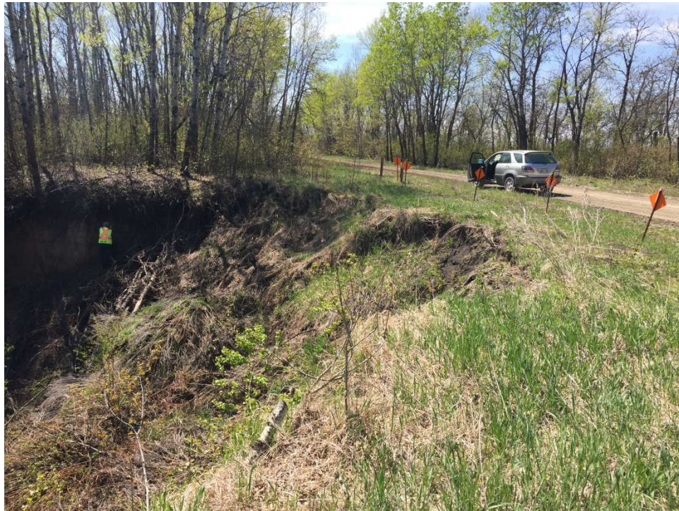
Photo 1 – Slope failure encroaching Road 54W at Site #94 (looking south).
