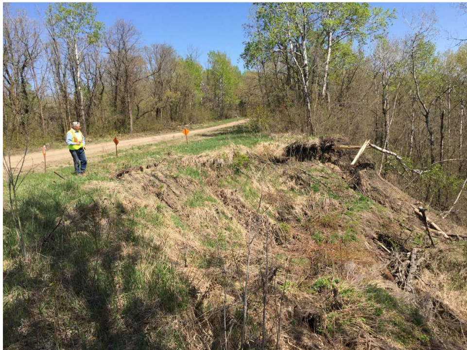
Photo 2 – Slope failure encroaching Road 54W at Site #94 (looking north).
