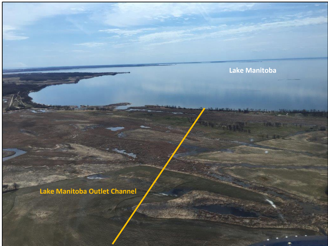
Photo 1. Approximate location of the Inlet of the Lake Manitoba Outlet Channel, looking southwest from approximately 14 U 5302187 E 5681941 N
